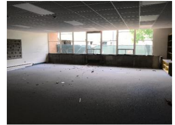
Classroom after demolition at Chestnut Hill
