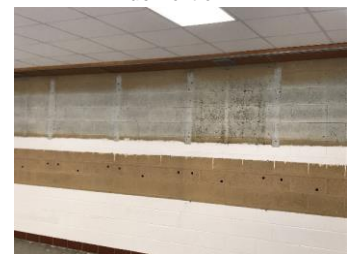
Drywall soffit at Siebert already being installed
